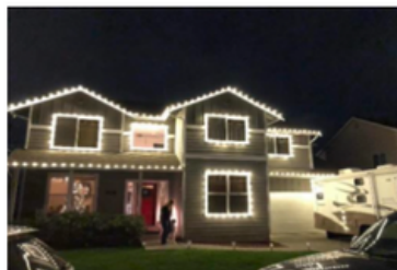
Windows, Garage Trim, and Fascia Boards Can Also Be Wrapped with Lights
